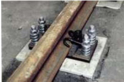
CRP on an underpoured socle
