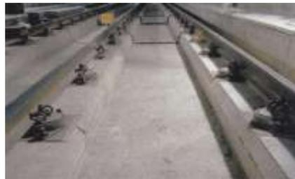
Cologne Egg, type CF1572 on concrete longitudinal plinths
